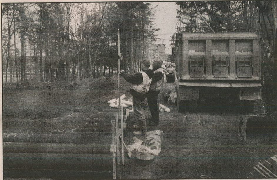
RICHARD MINGO and Robert Costa inspect Mingo's Presby Enviro-Septic pipe installation on property that has been acquired by the Redclyffe Restaurant in Robbinston specifically for the leach field installation.
